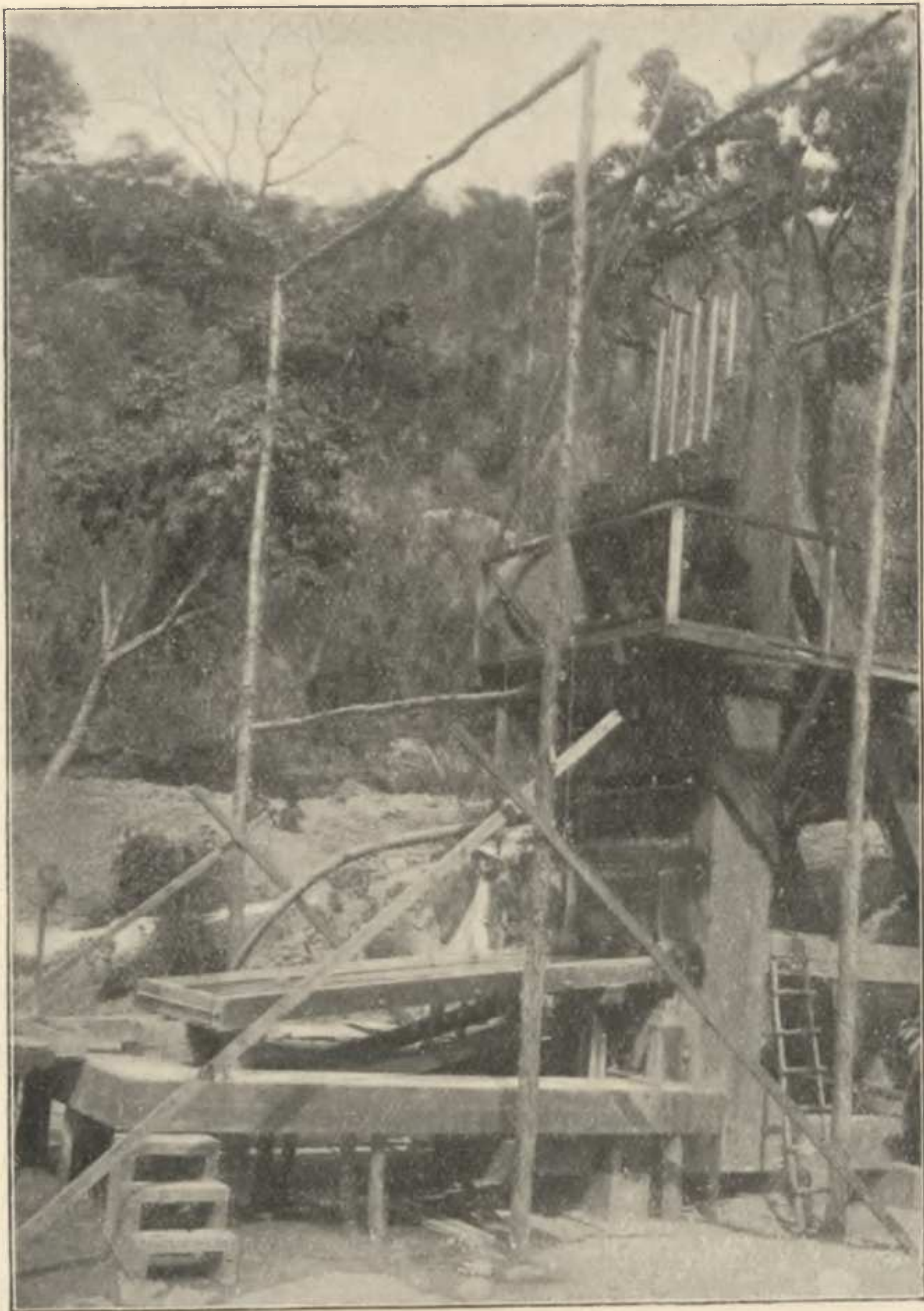
Five-stamp Battery, 1,250 lb. stamps, of Union Gold Mining Company, Ltd., on Wednesday Mine.
