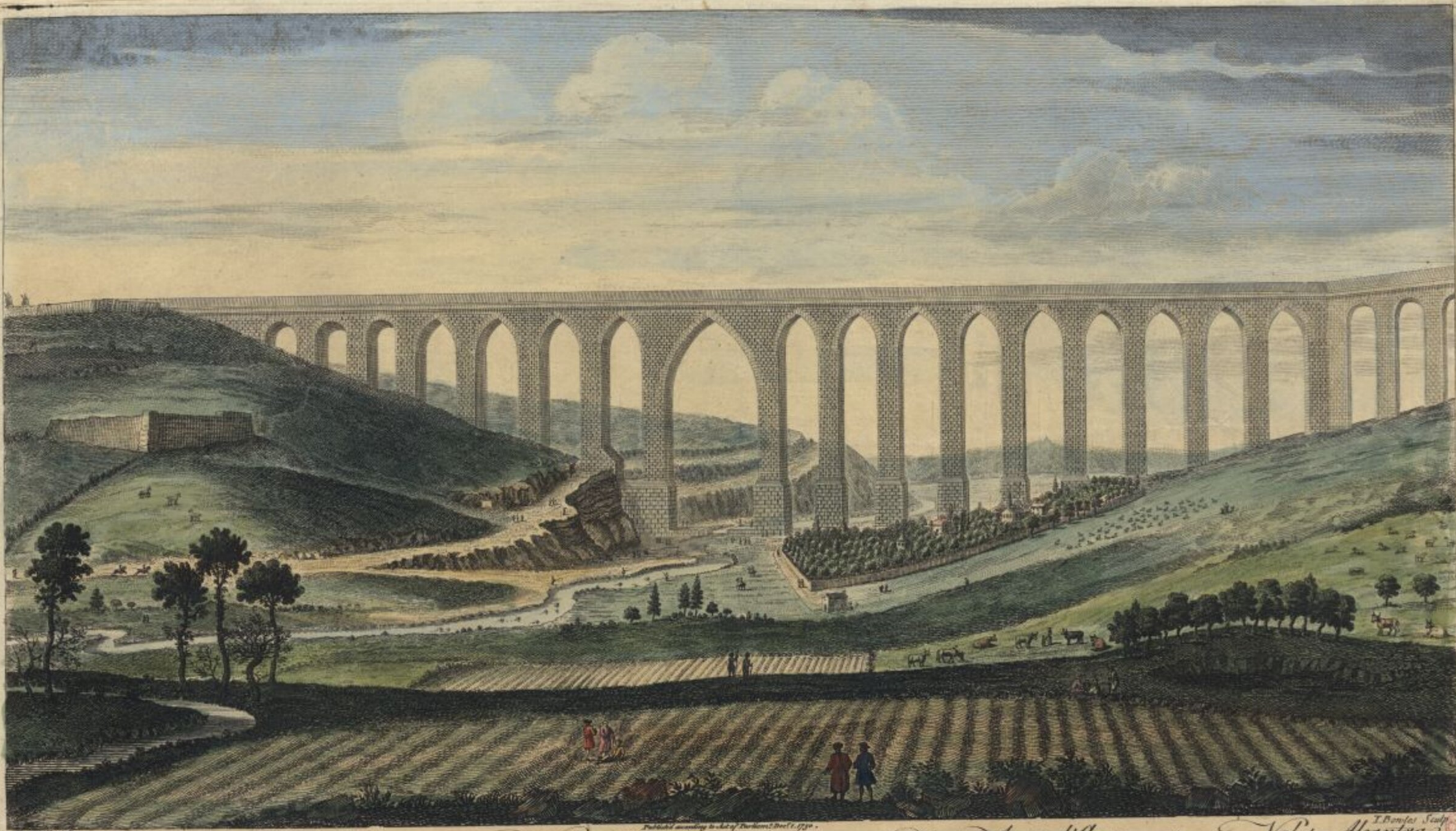
R. Black delin. A PROSPECT of the new Aqueduct of Lisbon, as Crossing over the Valley of Alcantra on Stone Arches, the Largest of which is 150 feet wide, and 249 feet High. Which is 47 feet higher than the Monument in London. PUBLISHED according to an Act of Parliament, Decr. 1739. PERSPECTIVA dos Novos Arcos d'Agua que a travessem o Val de Alcantra. altura do Mayor Arco he 332 Palmos, e a largura he 200 Palmos. I. Bonifas Sculp. London Printed for John Bowles at N. 13 in Cornhill.
