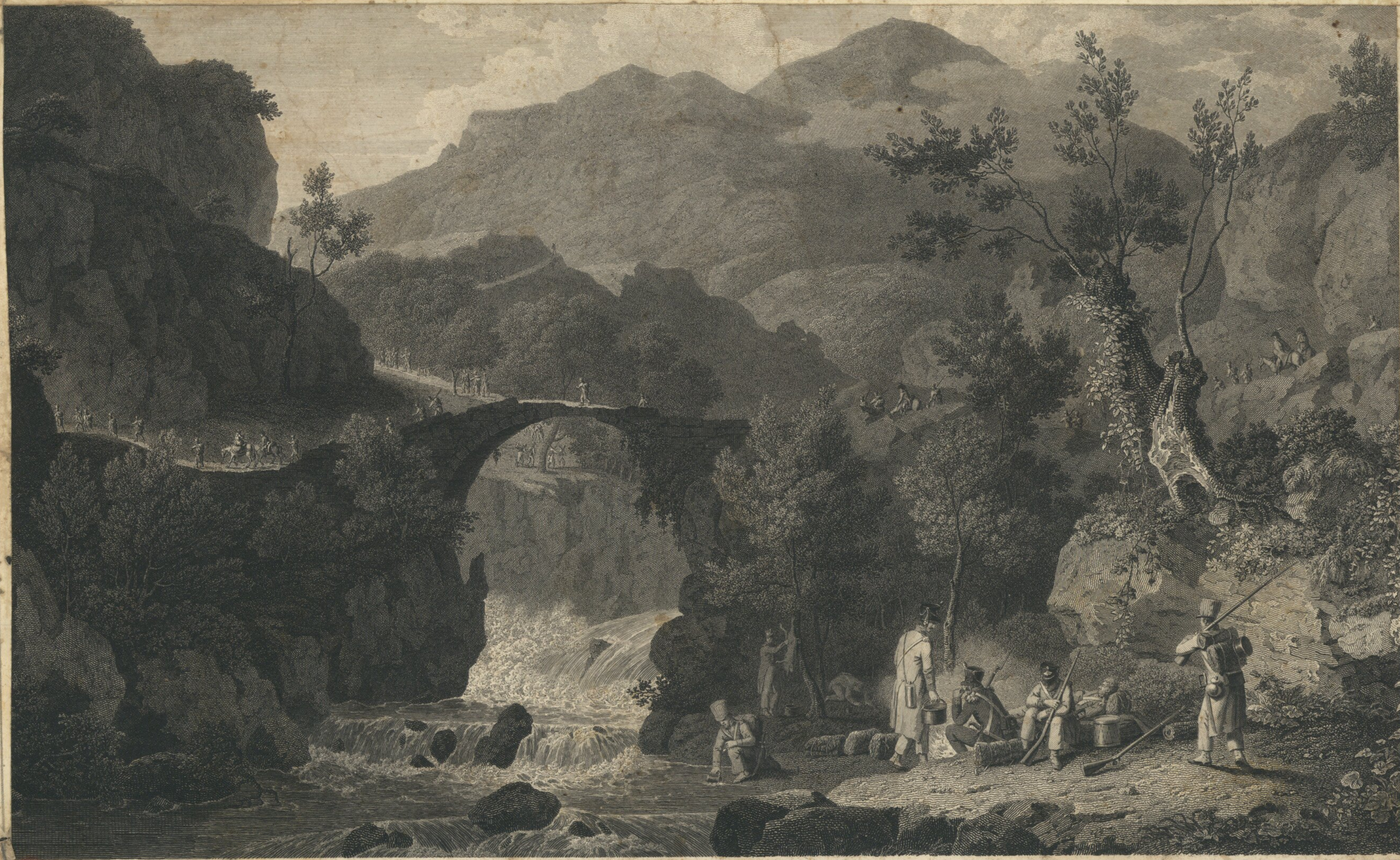
A VIEW OF THE BRIDGE OF MISERERE, ABOUT THREE LEAGUES FROM SALAMONDE.
