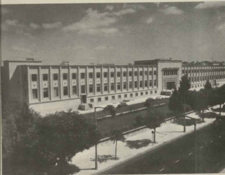
The National Civil Engineering Laboratory in Lisbon
